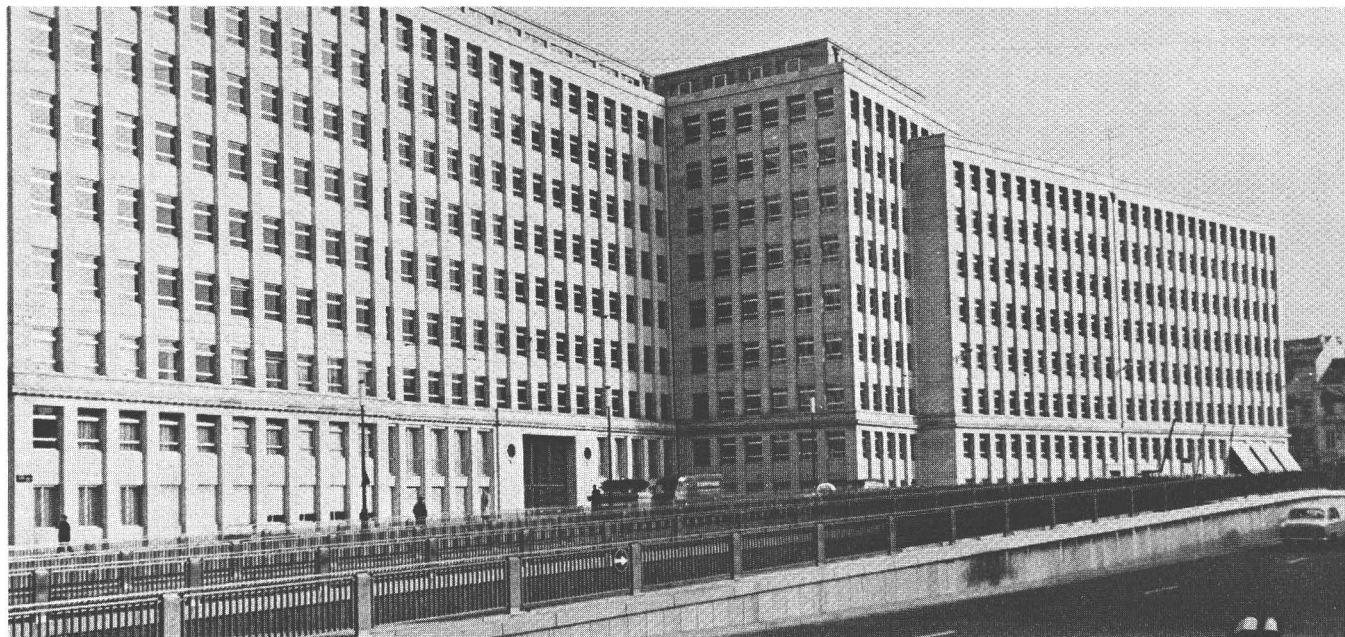
Negotiations for membership in the Common Market are being held in this new building in Brussels at 2 rue des Quatre Bras.
