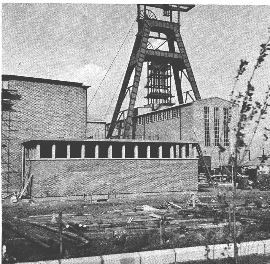
A new coal mine under construction at Noeuds-les-Mines, Pas de Calais
