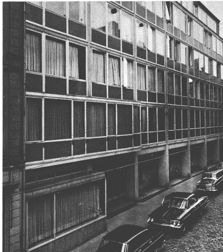
Court of Justice Headquarters: Cote d'Eich Street, Luxembourg.
