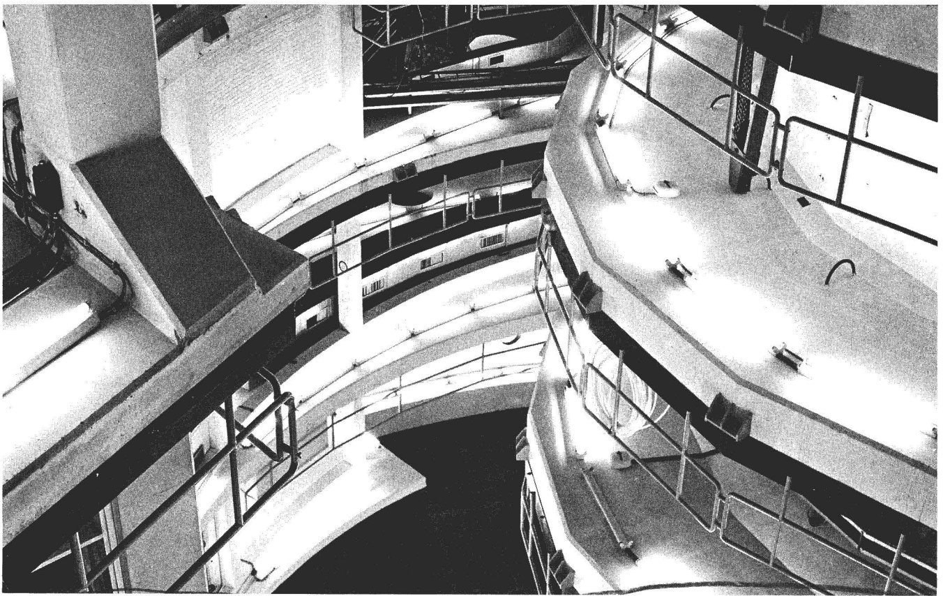
White concrete encircles the BR 2 reactor and instruments for its operation at Mol, Belgium. The high-flux materials testing reactor is operated jointly by "Centre d'Etude de l'Energie Nucléaire" (CEN) and Euratom.
