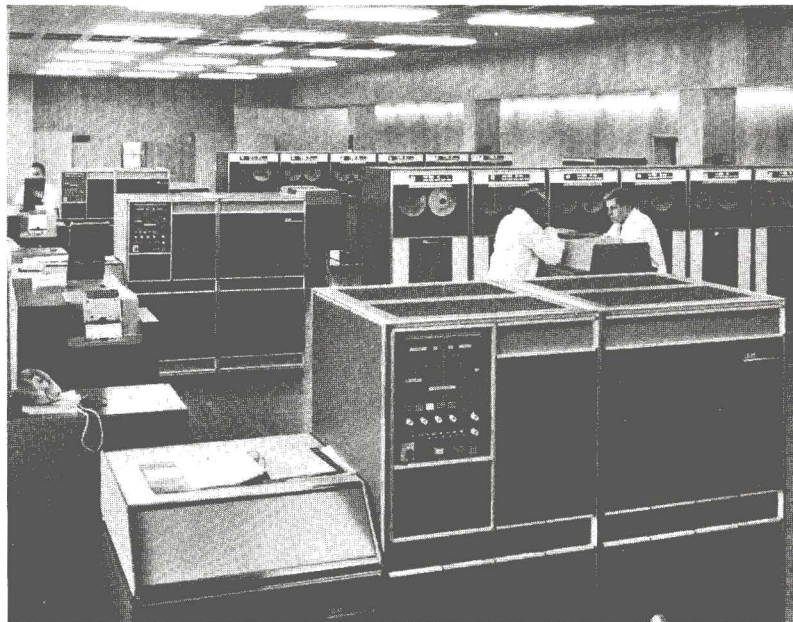
Data processing center of the Kundenkredit Bank KGAA, Düsseldorf, Germany. PHOTO: IBM WORLD TRADE CORP.
