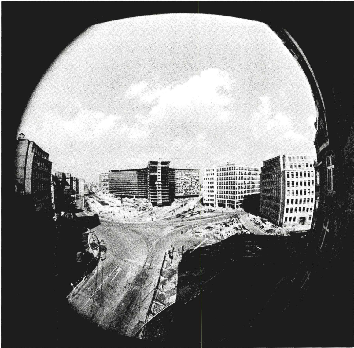
The European Community's new administrative center on the Rond Point Robert Schuman, Brussels. Last fall, the agriculture division moved into new quarters in the right wing of the building in the center. Other parts are rapidly nearing completion.
