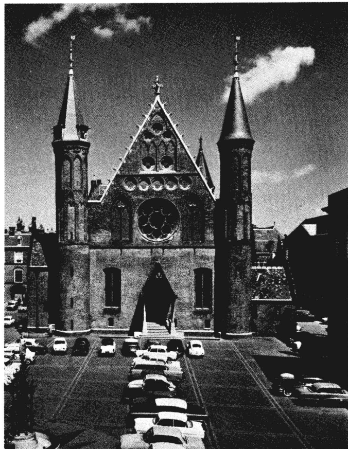
The Knight's Hall, the Hague, the oldest residence of the Counts of Holland, stands in the Inner Court, surrounded by the Houses of Parliament. It is the building used for all important state functions and the one in which the Queen opens Parliament each year. PHOTO: Courtesy of the Netherlands Information Service, New York. © Doeser Fotos, Laren.
