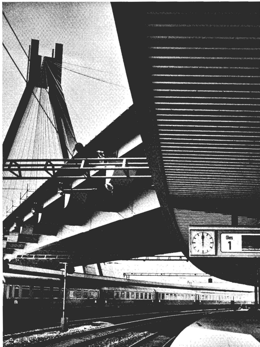
Luwigshafen Station, Germany. Solving the railroads deficits will be one of the most difficult tasks of the common transport policy. The beginning was made in 1969, when the Council of Ministers passed a regulation establishing some common accounting rules for railroads. At first, because of differences in accounting systems, the size of their deficits could not be compared, nor could the effects of state subsidies on competition be calculated.
