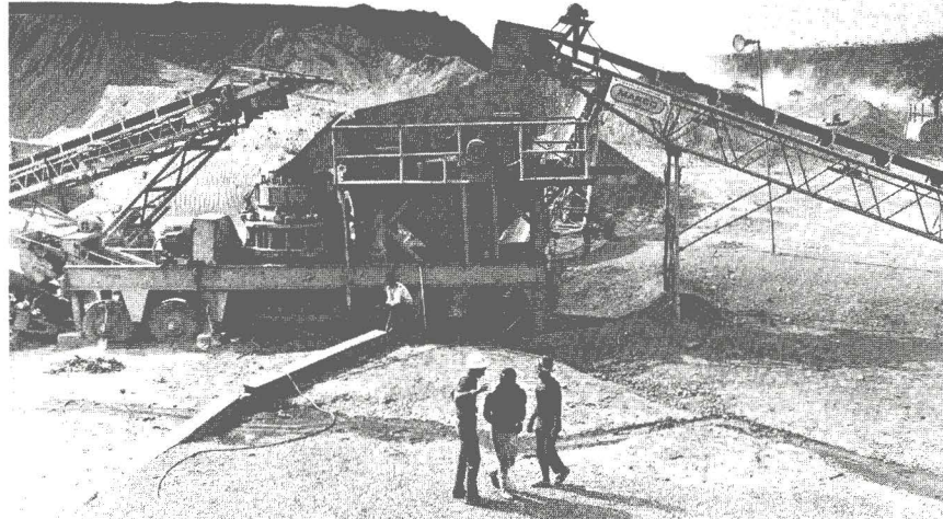
Roads such as the Tan-Zam Highway, linking Zambia's copper mines to the port of Dar es Salaam in Tanzania, are a prerequisite for industrial growth.
