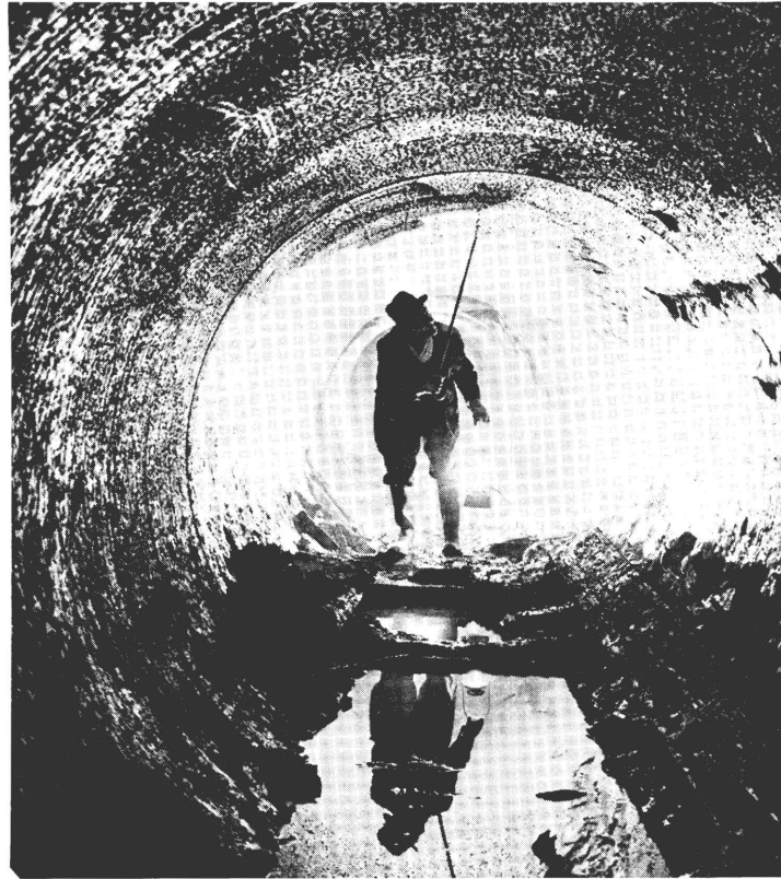
The pilot tunnel built a mile into the Channel near Dover, England, in the 1870's.
