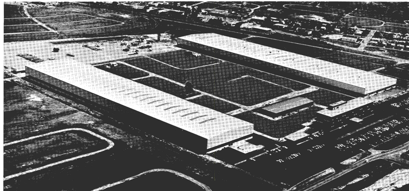
The German firm of Liebherr of America, Inc., recently built this plant in Newport News, Virginia, to manufacture hydraulic excavators.
