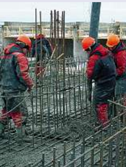
Wastewater Treatment Plant, St Petersburg, Russia
