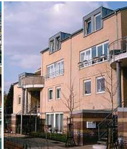
Flemish Housing Corporation, Belgium
