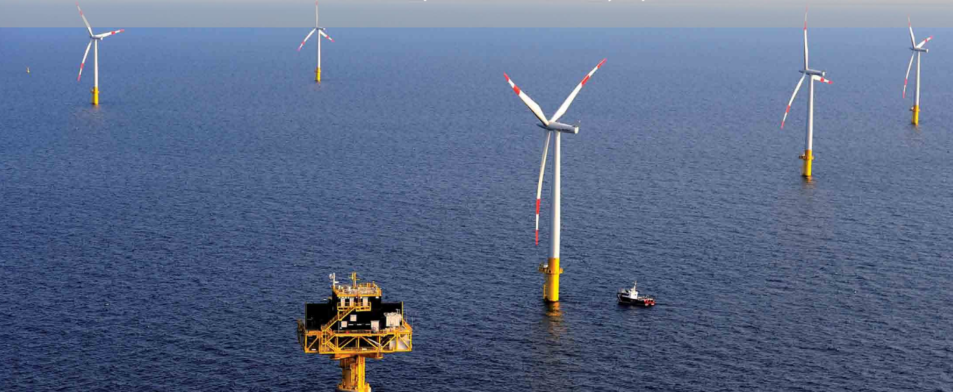
ENBW Baltic 1 wind farm, Germany
