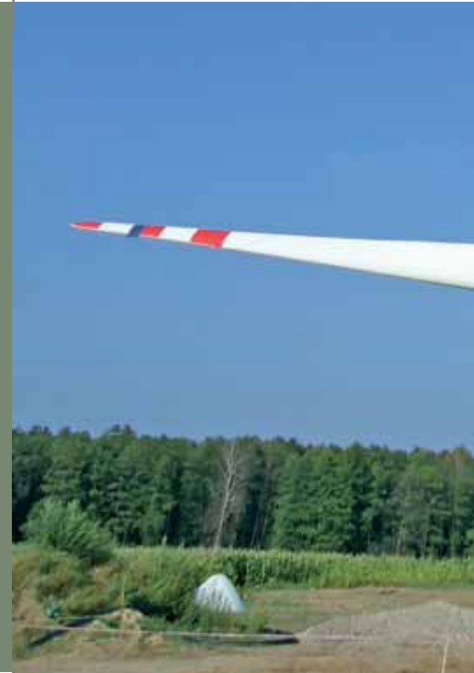
Golice Windfarm in Poland, JASPERS project
