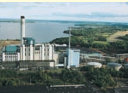
Combined heat and power plant in Västerås
