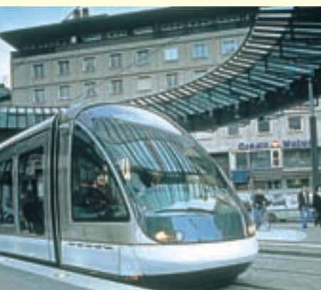
Strasbourg tram system
