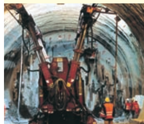
Bologna - Florence high-speed rail line
