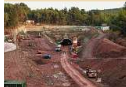
Construction of section of Prague-Dresden motorway
