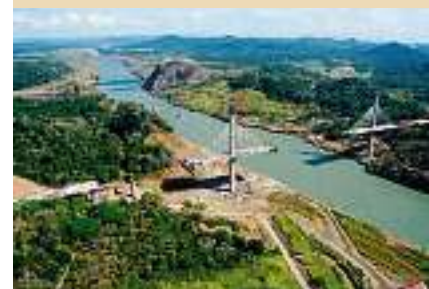
Bridge over Panama Canal
