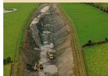
Construction of section of M4 motorway
