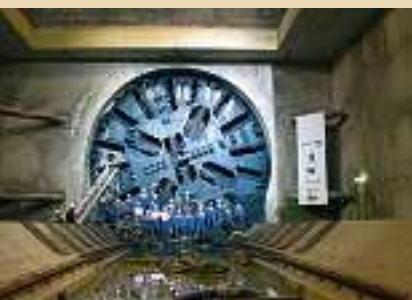
Tunnel-boring machine, site of A86 motorway
