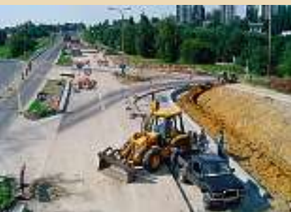
Rehabilitation of roads
