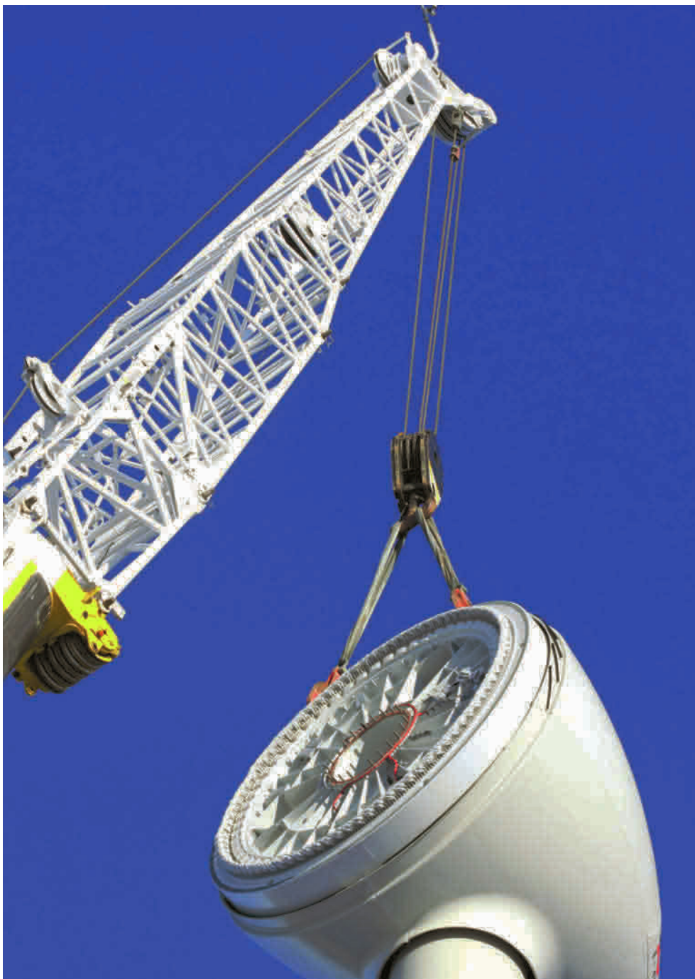
Construction of wind farm
