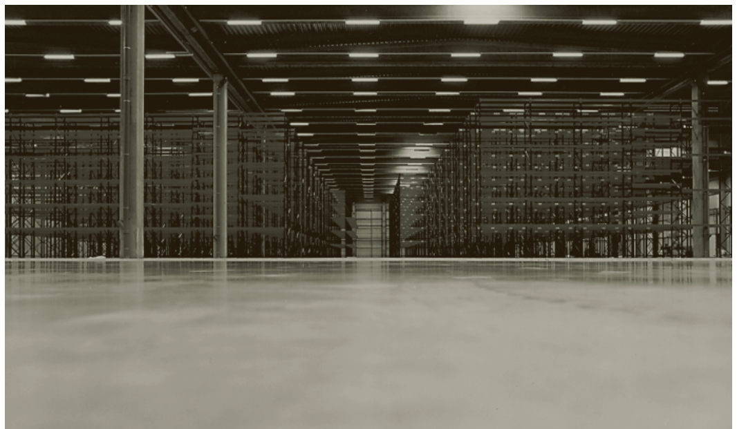
Construction of logistics facilities, Romania
