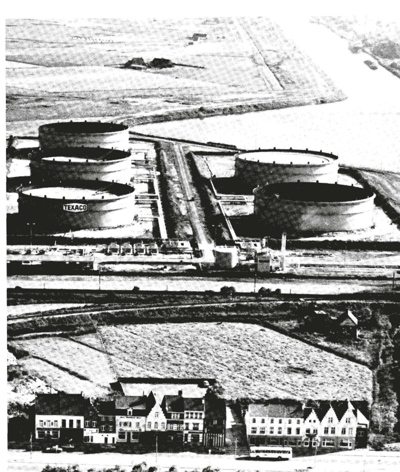
A new Texaco marine terminal at Zeebrugge, Belgium.
