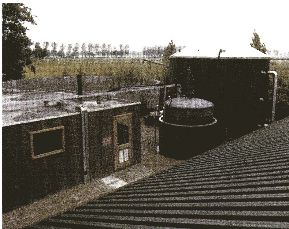
Picture 1: View of the original Pilot Plant in Duiven
