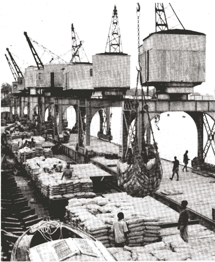
Electrification of cranes on the Lomé wharf was financed in part by the European Development Fund.
