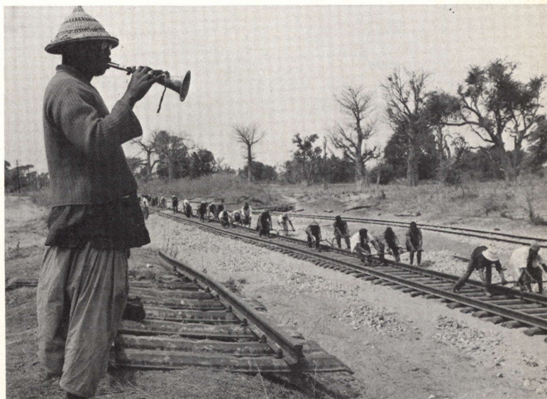
EC development funds helped repair this railway in Senegal.
