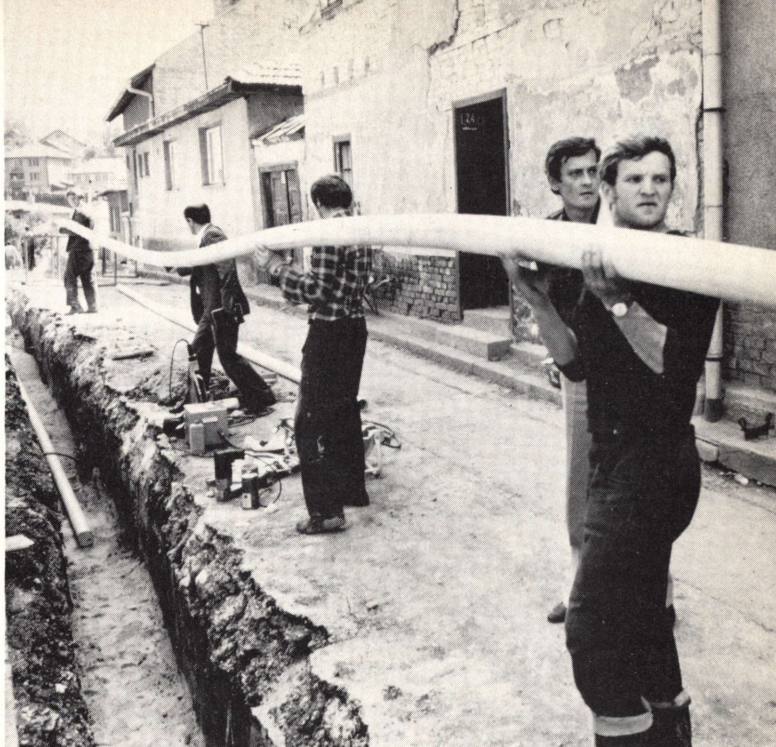
Yugoslavia is now facing the same problems as its European neighbors. Here, the city of Sarajevo converts to natural gas in order to fight air pollution. World Bank photo by Yosef Hadar
