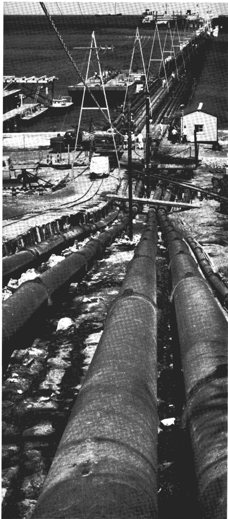
Venezuelan oil pipeline connecting to waiting tankers. © Cornell Capa, Magnum
