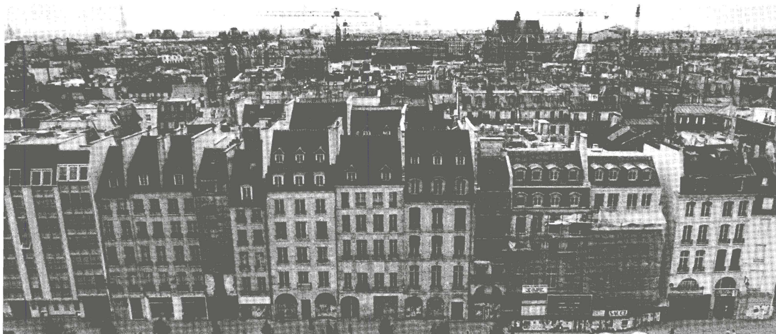
Evidence of the construction boom in Paris can be seen in the background of this view of old Paris, taken from the ultra-modern Georges Pompidou Center of Modern Art. © Jean-Pierre Laffont, Sygma
