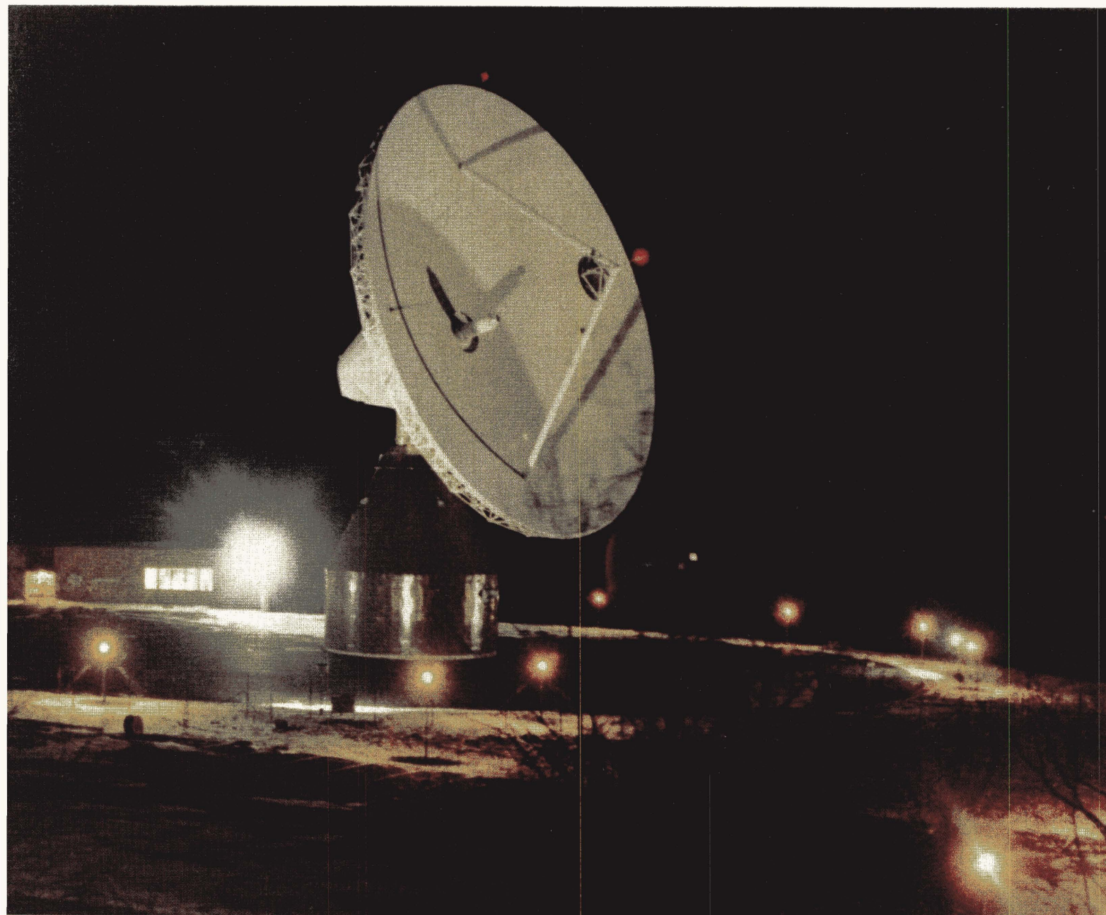
INTELSAT receiving dish in Sweden. Courtesy of INTELSAT
