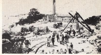
Sinking an operational shaft for Chunnel construction at St. Margaret's Bay on the Kent Coast in the 1870s.
