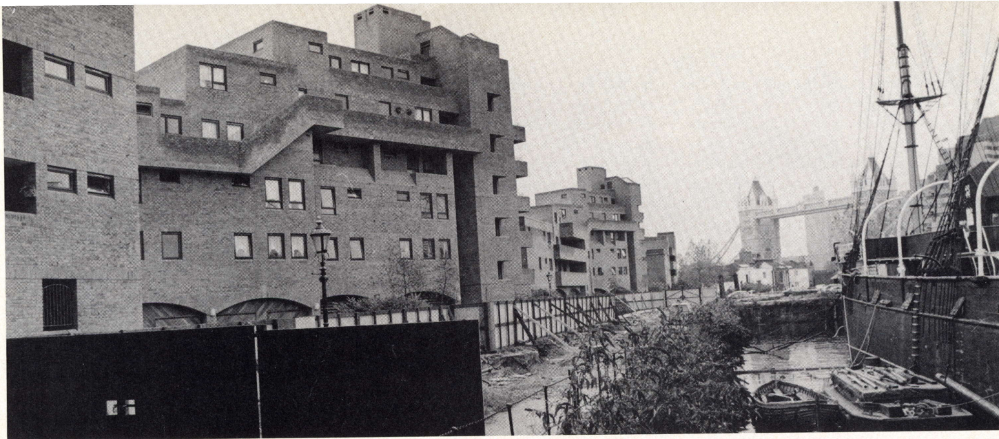
The old St. Katherine's docks, below the Tower of London, where some warehouses have been turned into luxury apartments. ©Keystone
