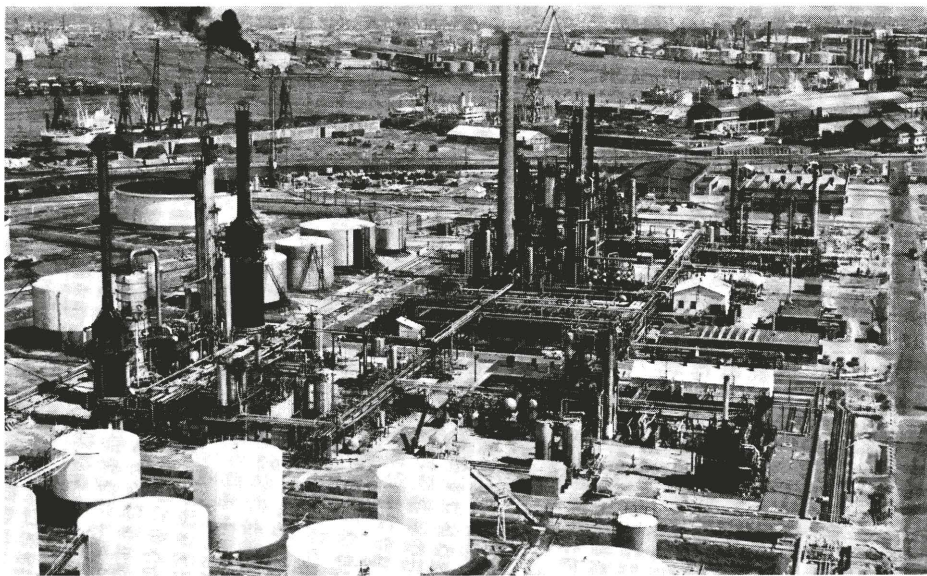
Shown here is a petroleum refinery in Antwerp, Belgium's largest port.
