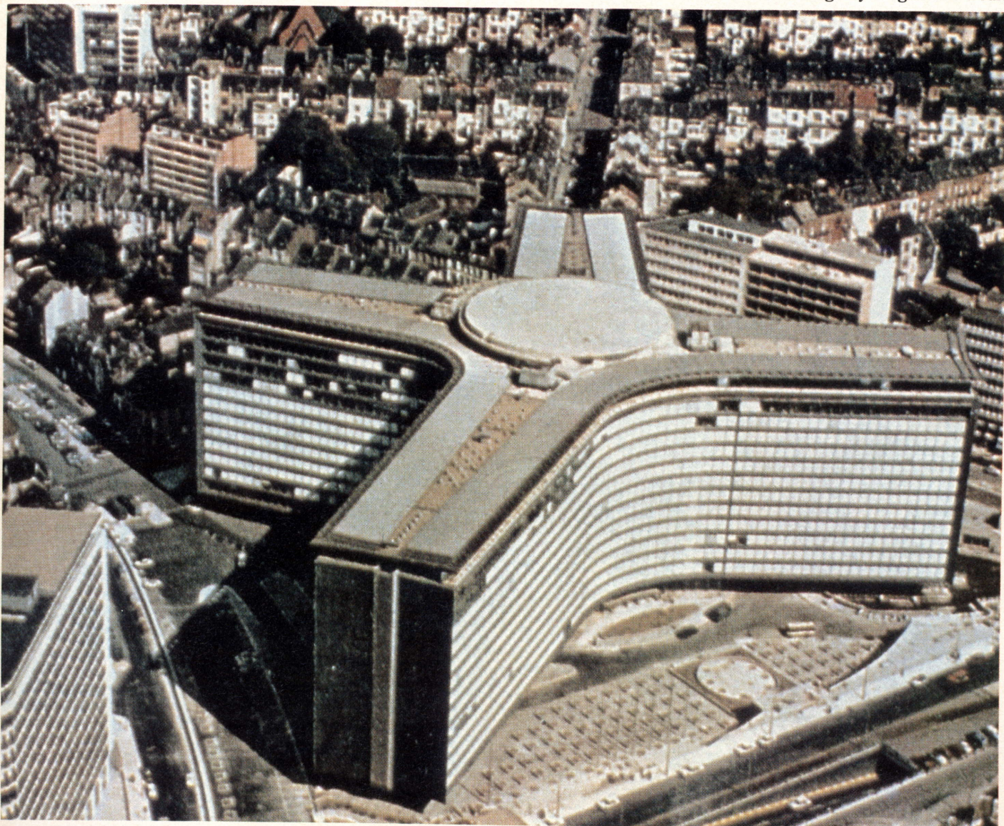
The E.C. Commission is housed in this building, known as the "Berlaymont," in Brussels.
