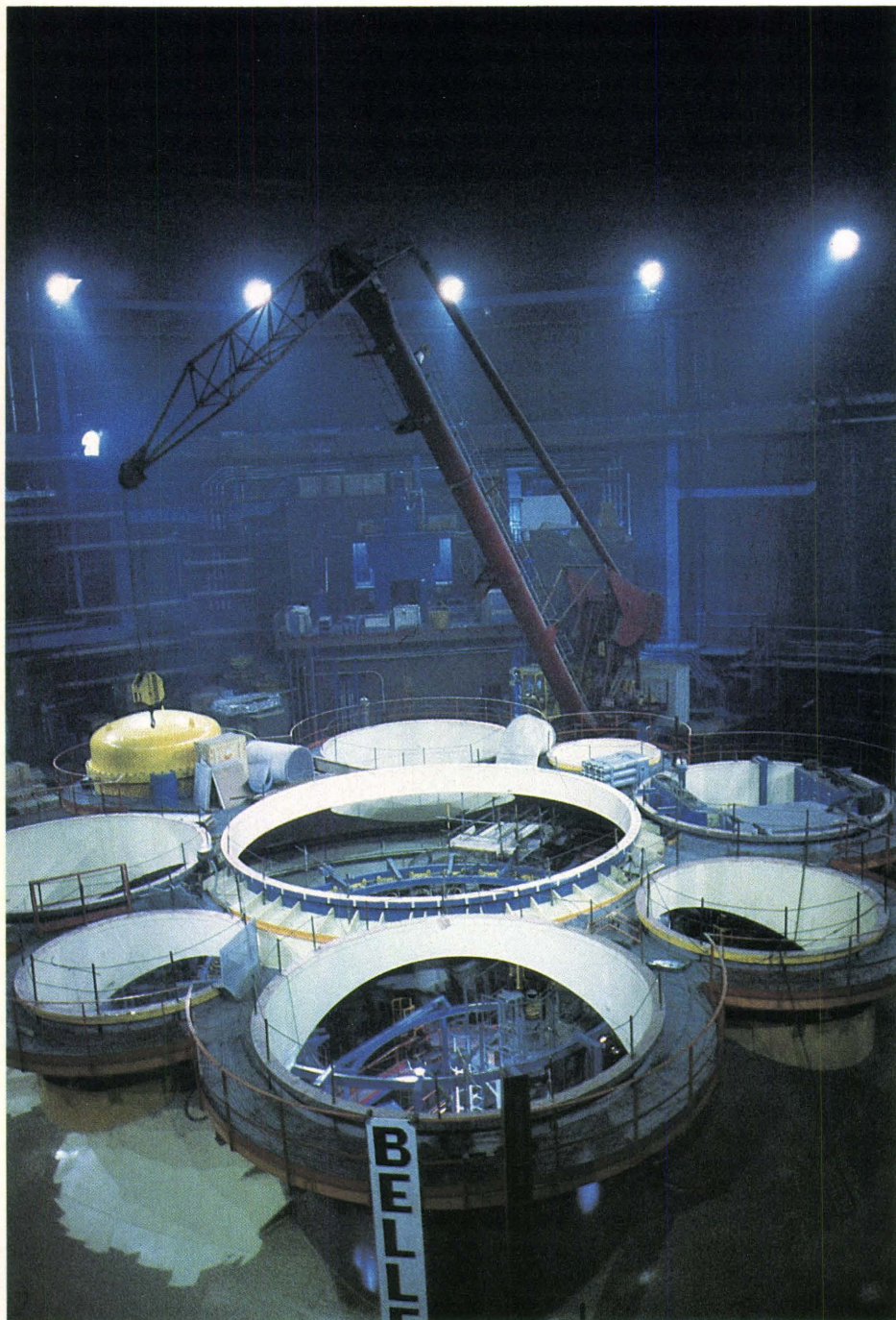
Inside the Superphénix reactor in France. Western Europe now obtains more than one-third of its electricity from nuclear power.
