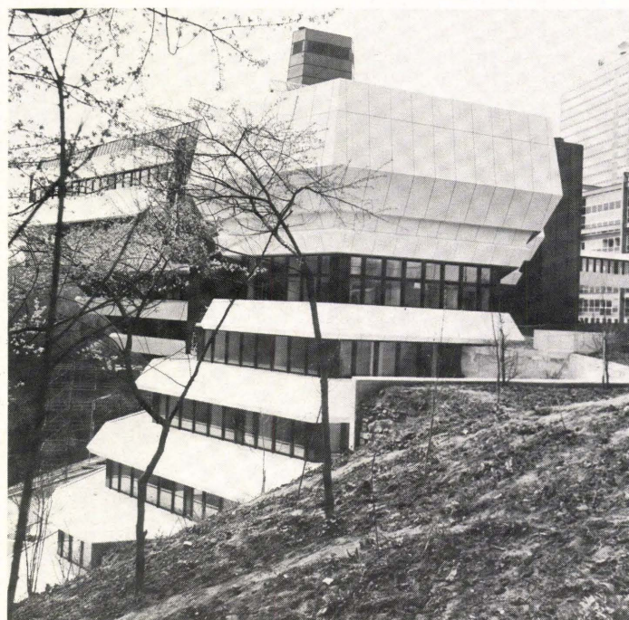
Luxembourg authorities hope that the ultra-modern building originally intended to house the European Parliament's sessions will now attract business conferences.
