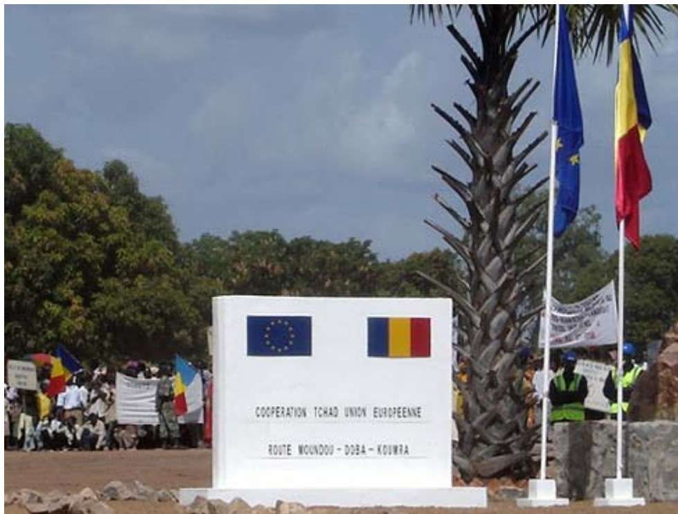
Bitumage de la route Moundou – Doba – Koumra
