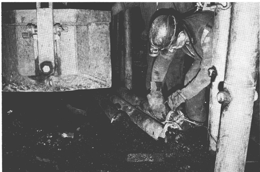
Fig. 37 - Loading of props and caps into the haulage rope trough
