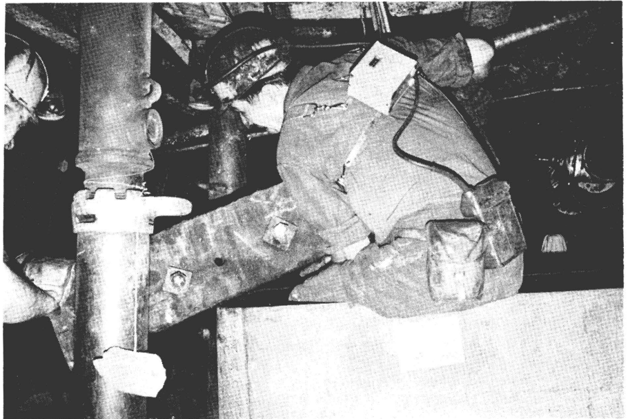
Fig. 40 - Reloading of ties
