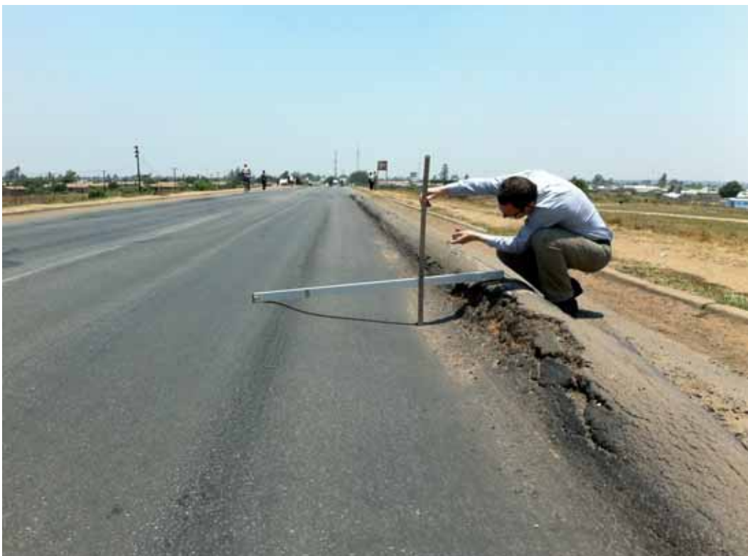
Road inspection in Tanzania
