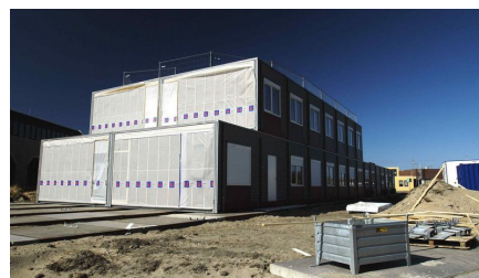
Temporary offices during construction
