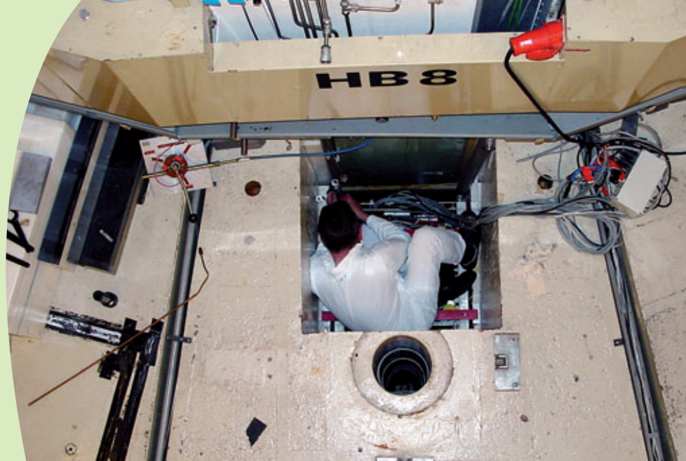
Figure 39 - Refurbishment of HB8
