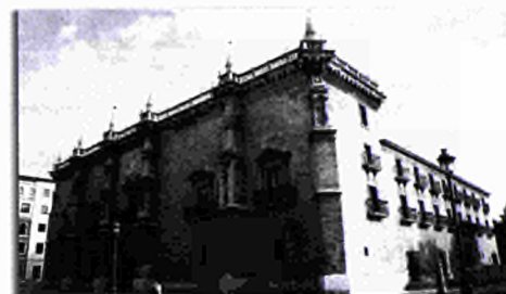
The restoration of the Santa Cruz Palace's facade in VALLADOLID includes testing the use of laser technology in rehabilitation work.
