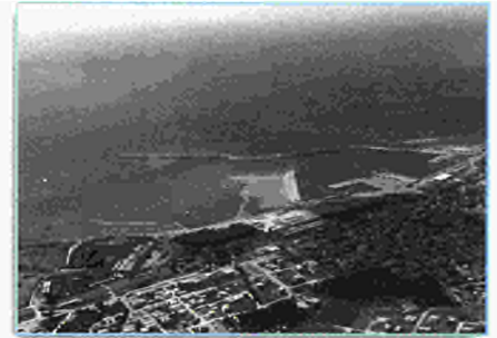
The Alexandroupolis POLI-NET project involves the restoration of an old building into an International Information Centre which will specialise in economic development activities with Balkan and Black Sea countries, harnessing new information technologies to develop networks for local businesses. It will also include a recreational and educational cyber café, and will thus help to increase local residents' knowledge and awareness of information technologies.
