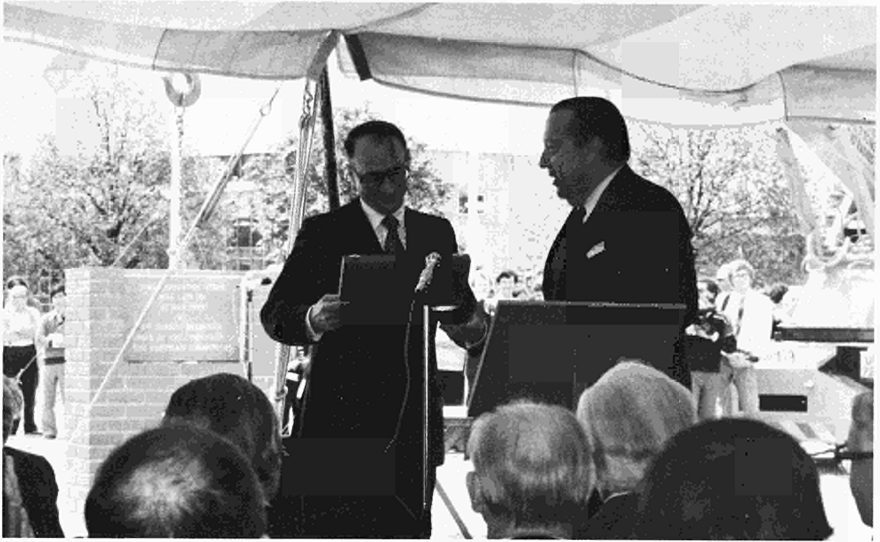
Fig.6 The Director of the Project (H-O Wüster) presents a silver trowel to Dr. G. Brunner (Member of the Commission of the European Communities responsible for energy, research, education and science) after the latter had laid the foundation stone of the main building of the JET Laboratory.
