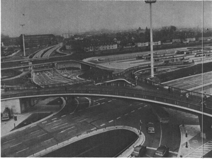
Fig. 7 - Star-shaped footbridge, Leverkusen
