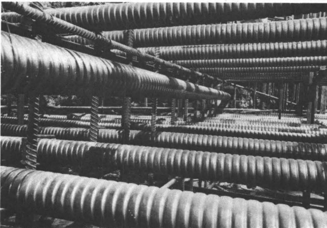
Fig. 5 The layers of 1\frac{1}{4} in. prestressing bars
