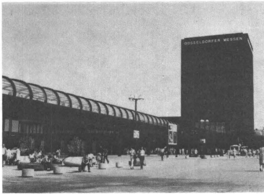
Fig. 17 - Enclosed footbridge complex at the new fair and exhibition site, Düsseldorf
