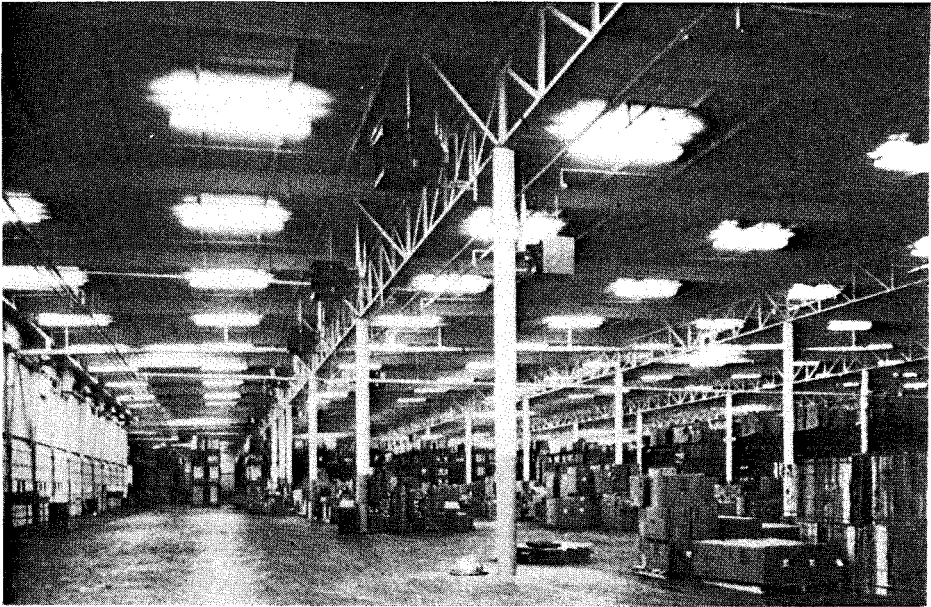
Figure 4. All-Steel Industrial Roof System
