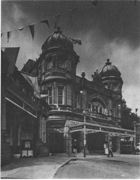
Fig. 1-The opera house restored
