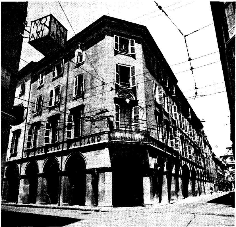
Fig. 12 : Building at Modena: view of the edifice during rebuilding.
