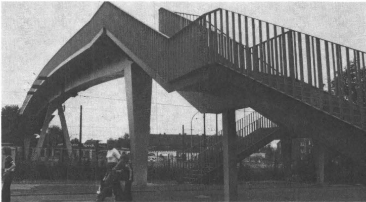
Fig. 3 - Footbridge in Essen (1976 after rebuild)
