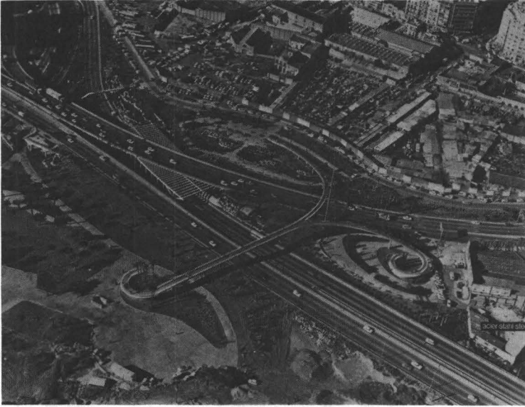
Fig. 28 - Suspended footbridge, Barcelona
