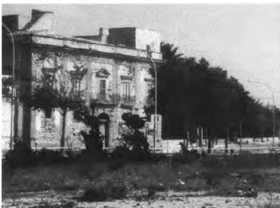
Fig. 7 Hopps Palace before the last restoration
