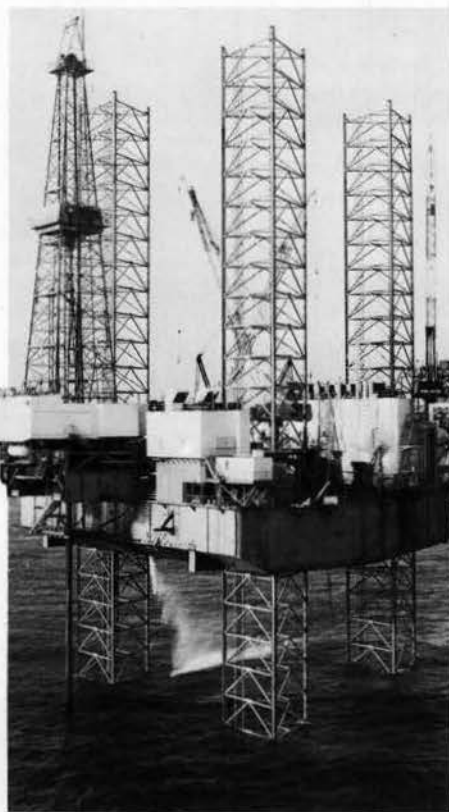
Apollo II – drilling for gas off the Lancashire coast.
