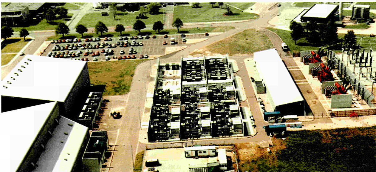
Fig.9 Outdoor high voltage power supplies for neutral beam and radio frequency heating systems
