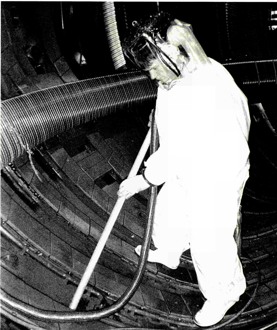
Fig 8: Installed Beryllium tiles on the belt limiter. A suited worker is cleaning the vessel before operation
