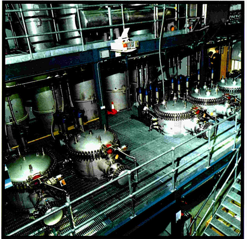
Fig.30: The Active Gas Handling System showing the five cryogenic forevacuum modules with buffer tanks and distribution system in the background.
