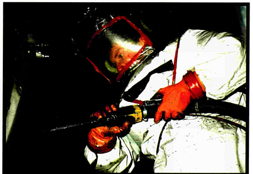
Fig.8: Cleaning the vacuum vessel walls
