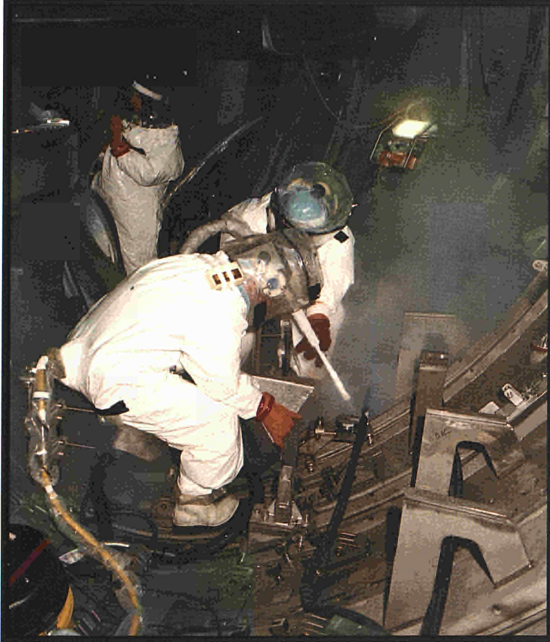
Fig.25: Carbon dioxide pellet blasting in the vessel
