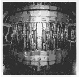
Fig.10: Reinforced ring installed inside the JET vessel;
