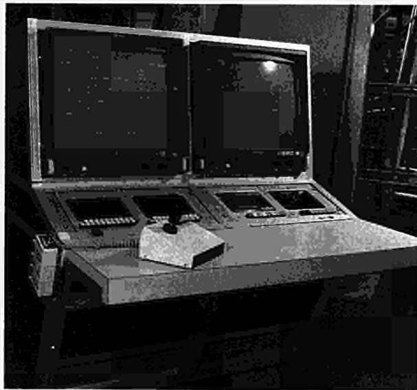
Fig.35 Remote handling work station.
