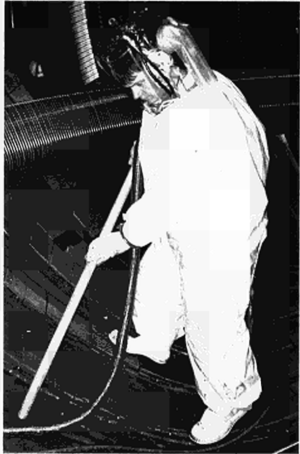
Fig 12: Installed Beryllium Tiles on the Belt Limiter. A Suited Worker is Cleaning the Vessel Before Operation.
