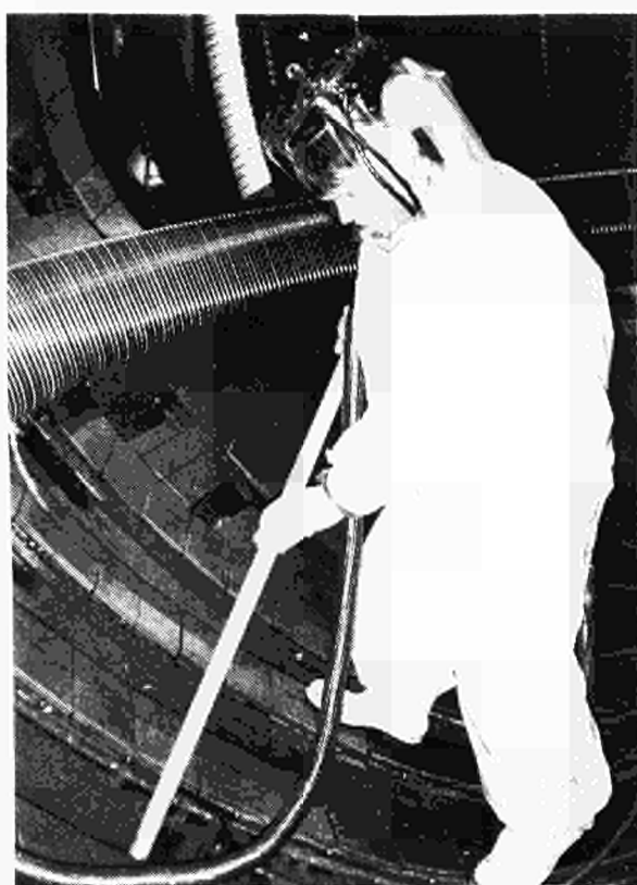
Fig. 5: Belt limiter during installation. Note the biological protection
