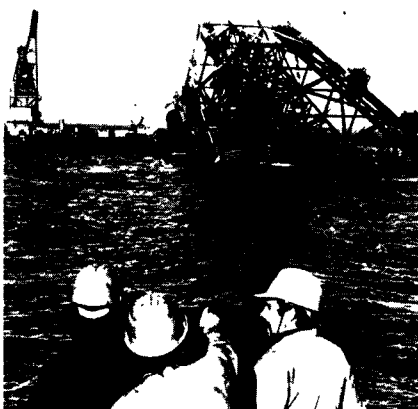
Oil production platform being positioned in the North Sea — but how long will the oil flow?
