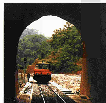
CFCO realignment: the long tunnel
