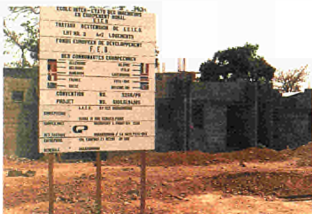
EIER extension: teachers' housing under construction ...
