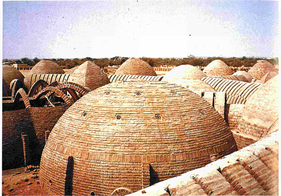
With its domed wards, Kaédi hospital is reminiscent of an African village
