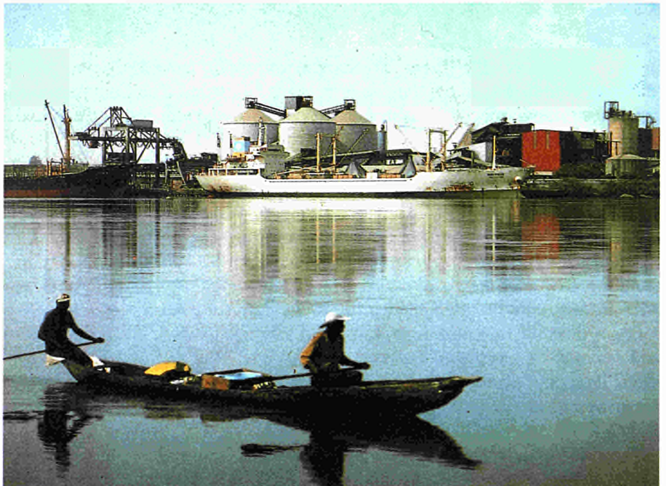
Douala cement works
