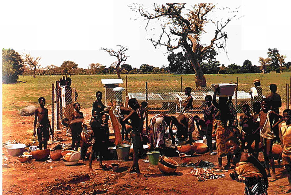
Solar pump for a Malian village
