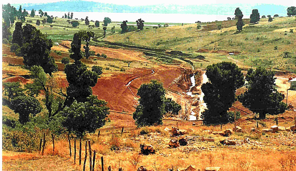
Tunnel outlet to Lake Finchaa
