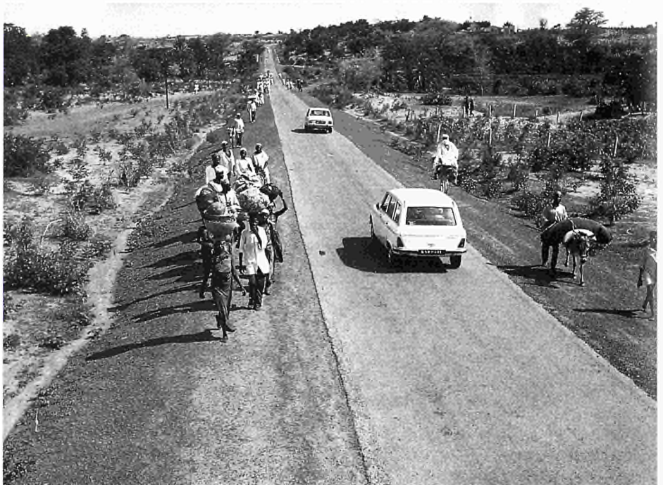
Widening the Zinder-Niamey road
