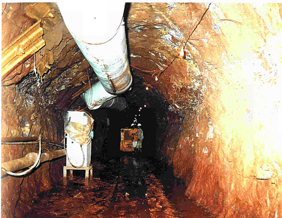
Amarti diversion tunnel under construction
